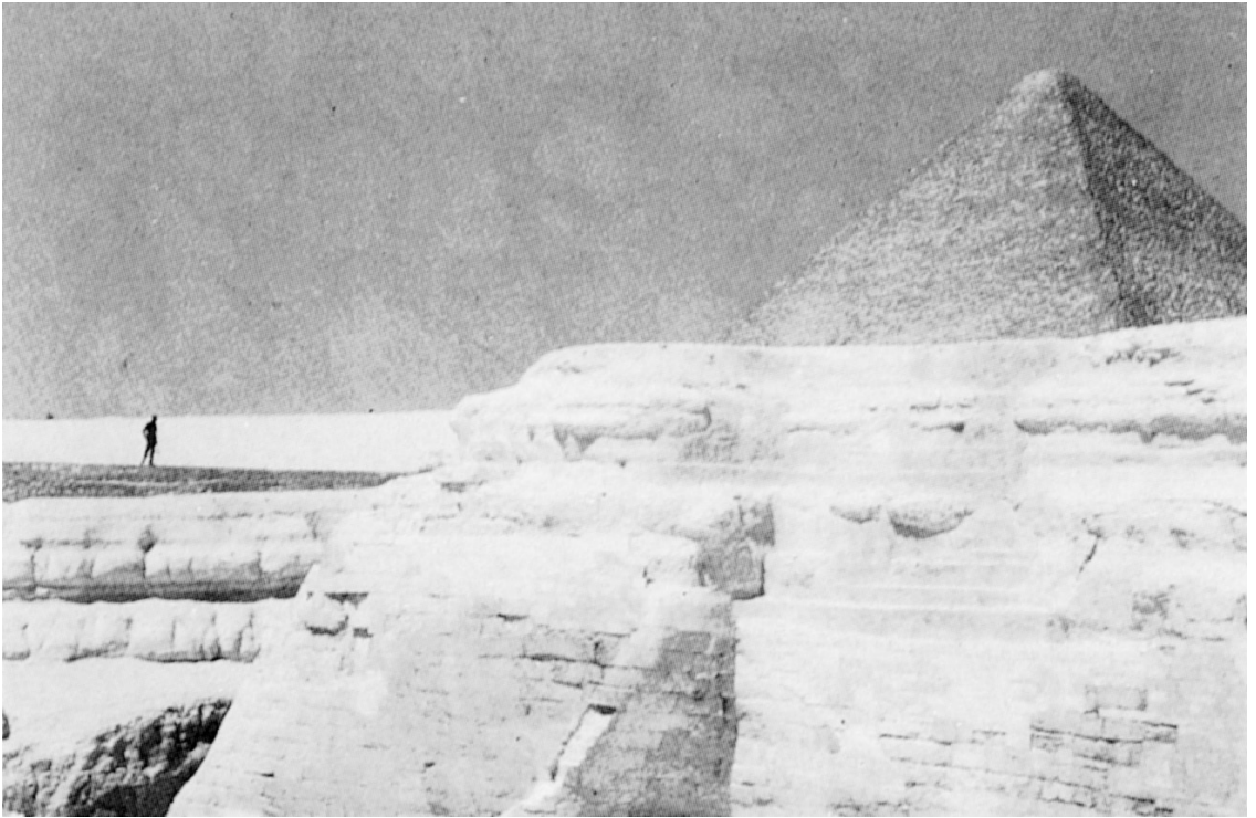
71 The rear of the pit or trench out of which the body of the Sphinx was carved again shows the characteristic vertical fissures and scalloped coves of precipitation-induced weathering. The rump of the Sphinx, also shown, has been partially covered in repair blocks in modern times.
