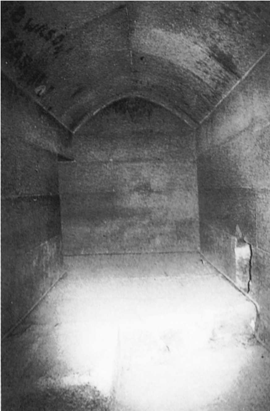
48 The lowest of the three chambers in the Menkaure Pyramid. Its ceiling, defaced with graffiti in modern times, consists of 18 huge granite slabs laid in facing gables, hollowed out from beneath to give the effect of a concave barrel vault.
